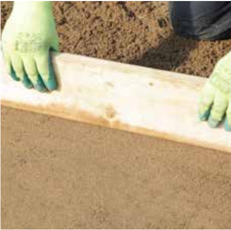
3. Screed out a 30-40mm sharp sand bed.
