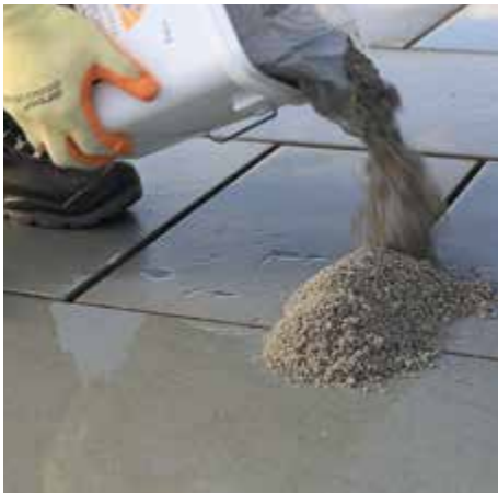
3. The Fast Point material is poured onto the paving
