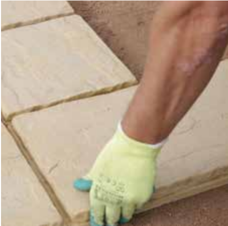
5. Make a solid connection when laying the NEXTpave to ensure a perfect uniform joint.
