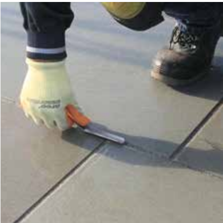
6. The joints are struck off using a pointing iron. Any gaps that are revealed are refilled with Fast Point.
