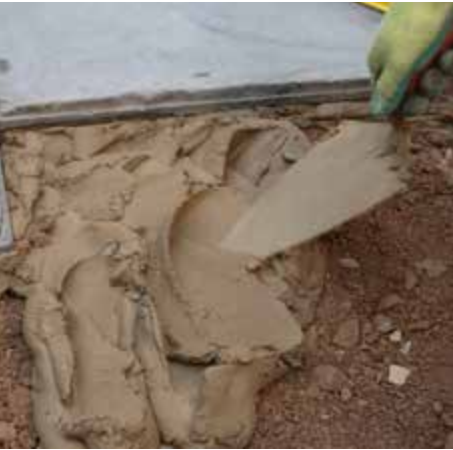
3. Install the engineered NEXTpave flags onto a full bed of mortar.
