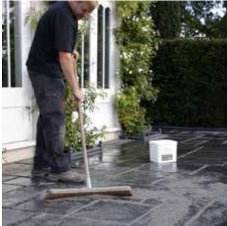
6. After 24 hours brush in Stonemarket FastPoint following the instructions on the tub, using plenty of water.
