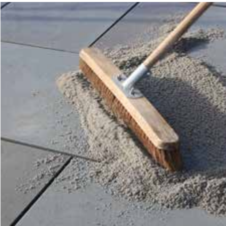
4. The material is brushed into the joints ensuring the joint voids are full
