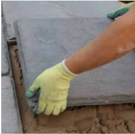
4. Install the engineered NEXTpave using the laying pattern.
