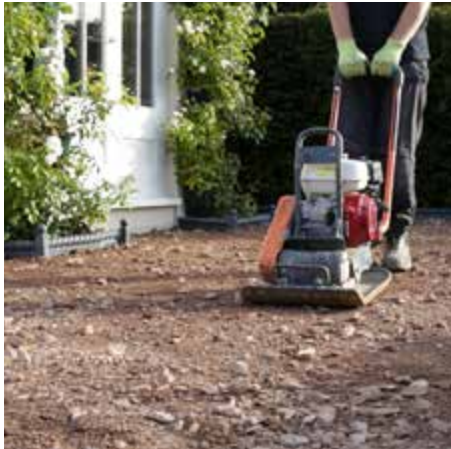
2. Prepare the ground as normal with compacted hardcore, achieving the correct falls for drainage.
