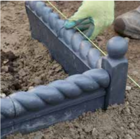
1. Install your choice of edge restraint on a concrete footing around the perimeter of the patio.
