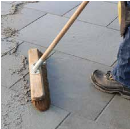
5. Any excess is carefully brushed off. Particles left on the paving may leave a speckled finish.
