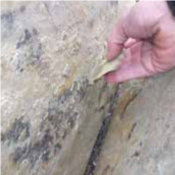
Surface delamination
