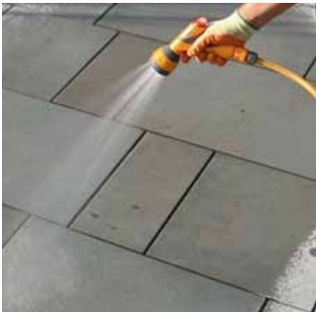
1. The paving is soaked with a hose. Keep wet throughout to avoid temporary staining.
