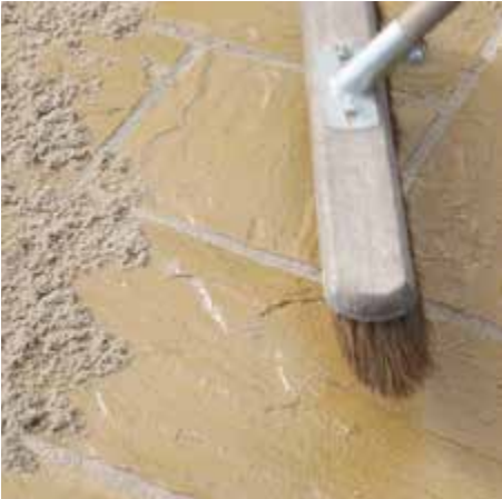
6. Brush in Stonemarket FastPoint following the instructions on the tub, using plenty of water.
